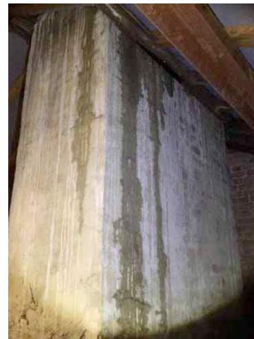
Top: leaking affecting adjacent ceiling as evident in roof void Centre: general external view of chimney Bottom: details of flashing
